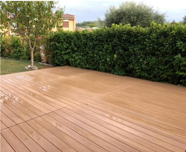
The laying of the aligned DECK boards (therefore NOT QUARTERDECK LAYING) is FORBIDDEN for SOLID TIMBY DECK DELUXE.
