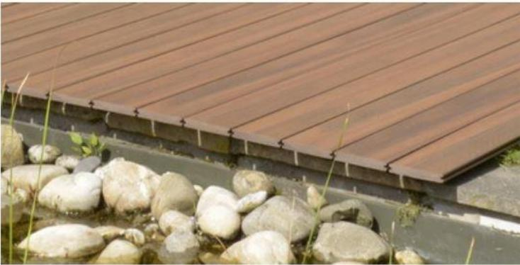
For a finishing aesthetically better it is possible to use an L-shaped profile, on the market, to lay on the deck, marking points on which holes must be made.
