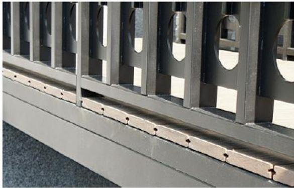
4B. With an L-shaped alluminium finishing profile.
